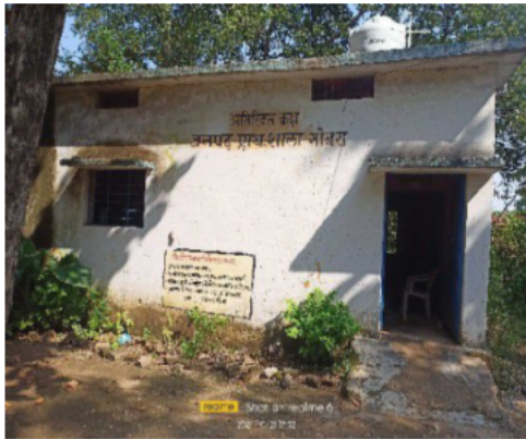
Polling Station Front View
