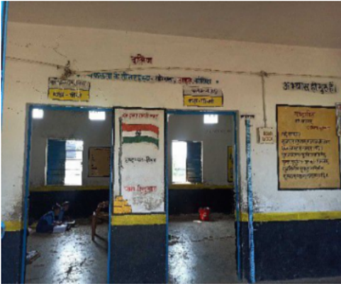
Polling Station Building Front View
