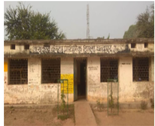
Polling Station Front View
