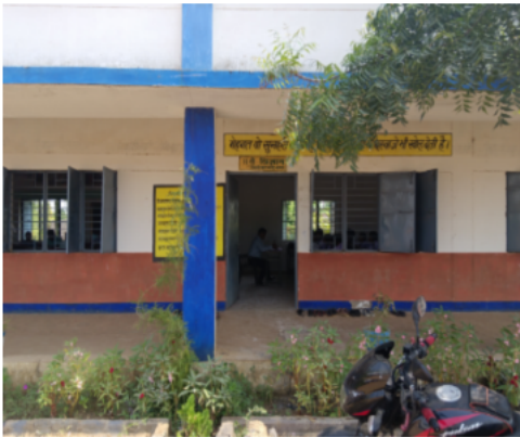
Polling Station Front View
