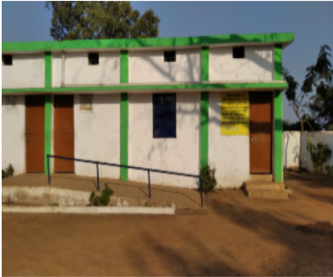
Polling Station Front View
