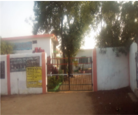
Polling Station Front View
