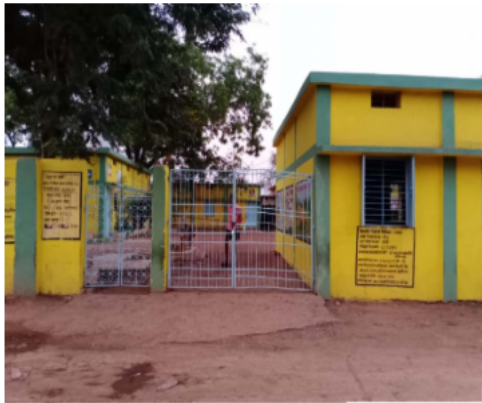
Polling Station Front View
