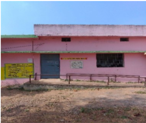
Polling Station Front View
