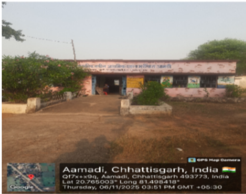
Polling Station Building Front View
