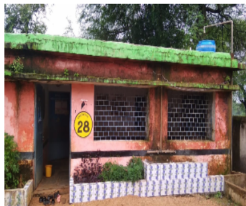
Polling Station Front View
