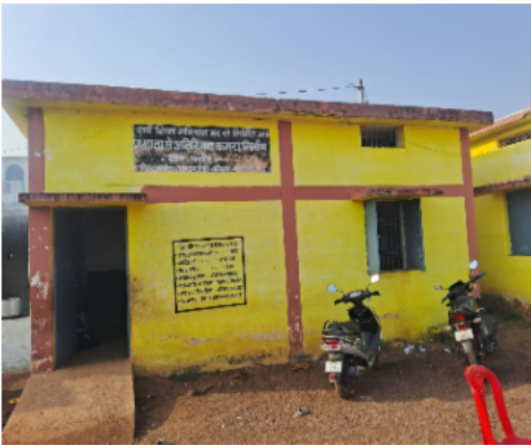
Polling Station Building Front View
