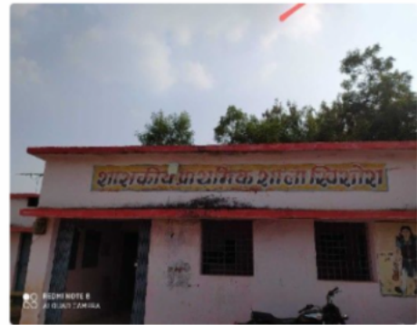
Polling Station Front View
