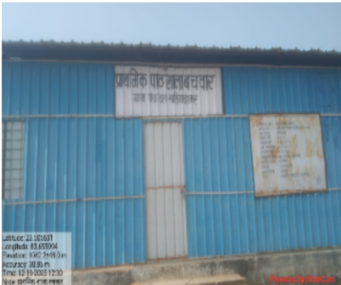
Polling Station Front View
