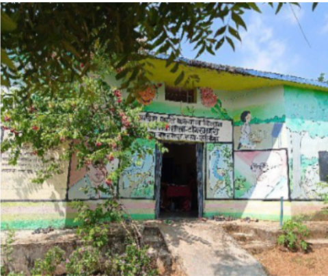
Polling Station Front View
