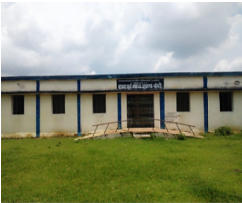
Polling Station Building Front View
