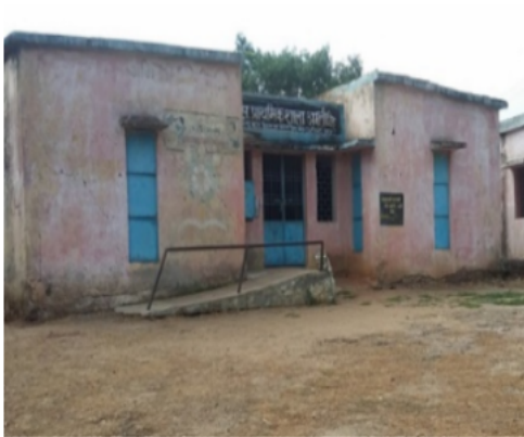
Polling Station Building Front View
