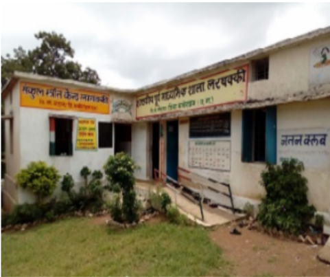
Polling Station Building Front View
