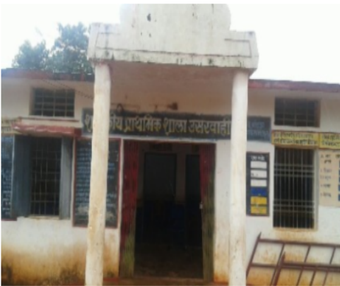
Polling Station Building Front View
