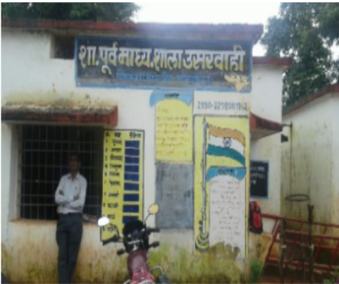
Polling Station Building Front View
