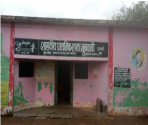
Polling Station Building Front View
