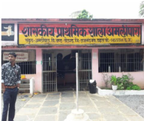
Polling Station Building Front View
