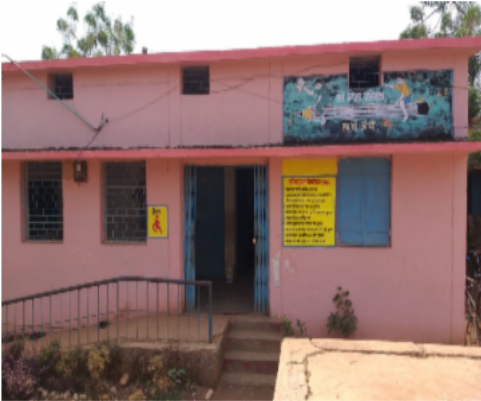
Polling Station Building Front View
