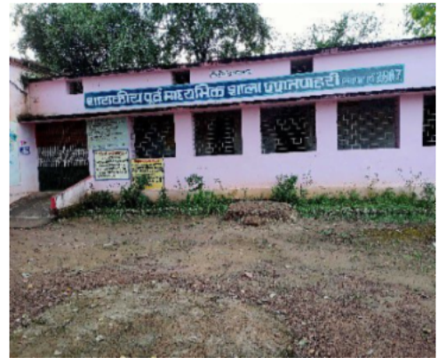
Polling Station Front View
