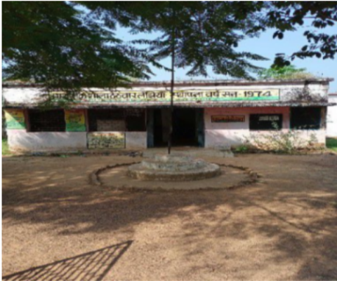
Polling Station Front View
