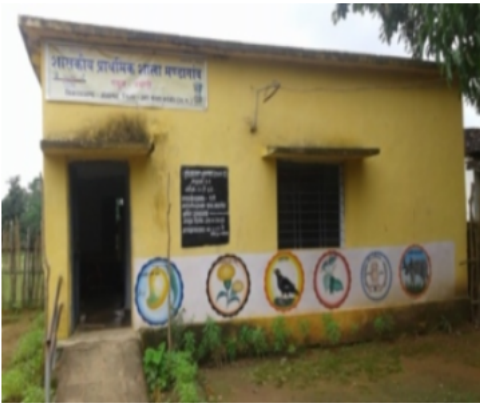
Polling Station Building Front View
