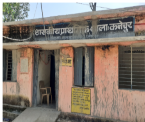
Polling Station Front View
