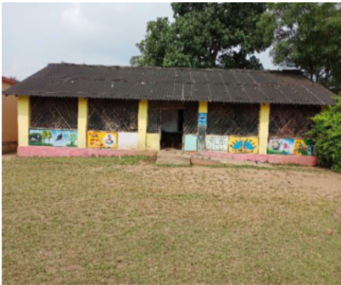
Polling Station Front View
