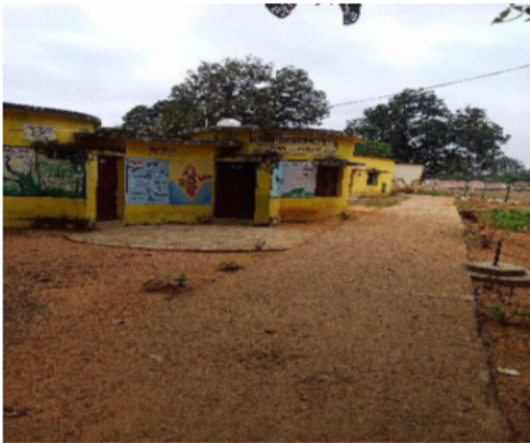
Polling Station Front View
