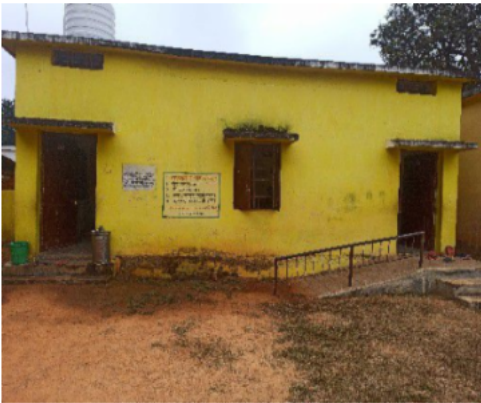
Polling Station Building Front View
