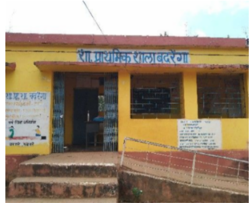
Polling Station Front View
