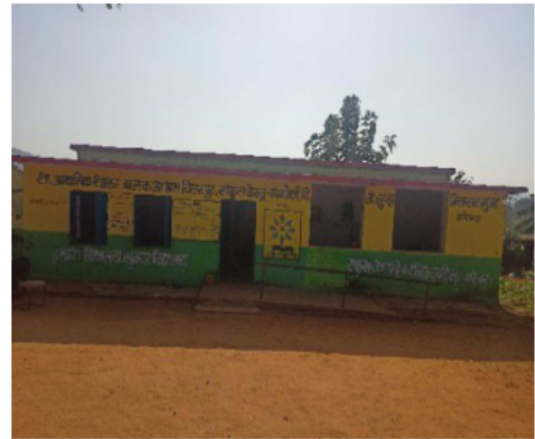
Polling Station Front View
