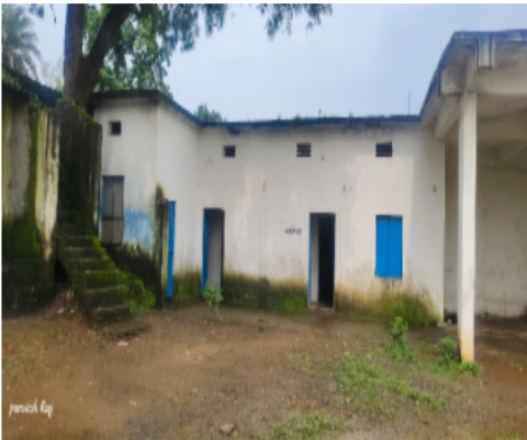
Polling Station Building Front View
