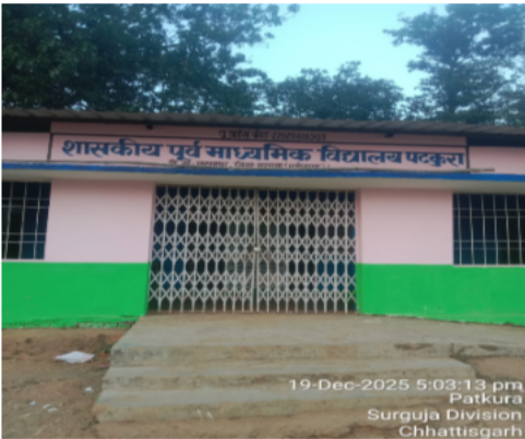
Polling Station Building Front View
