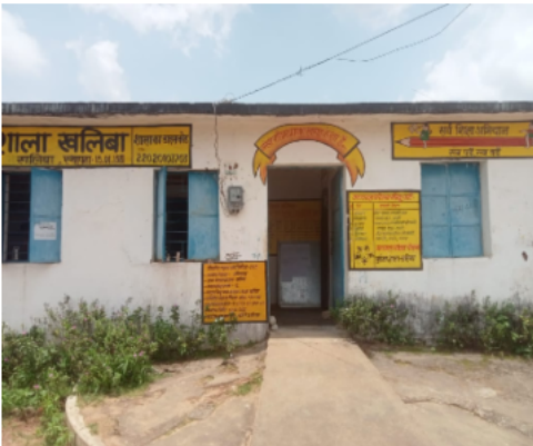
Polling Station Building Front View
