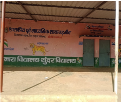
Polling Station Building Front View
